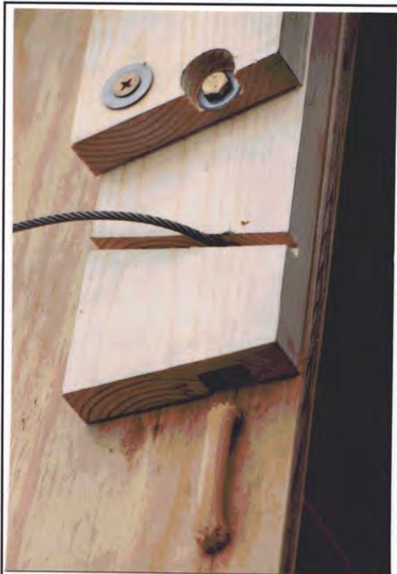
Figure 3: I constructed this model to display details of the basket base construction. You are looking down on the bottom of the basket. The plywood is the basket floor and the two skid plate layers are cross-sectioned to show details.
